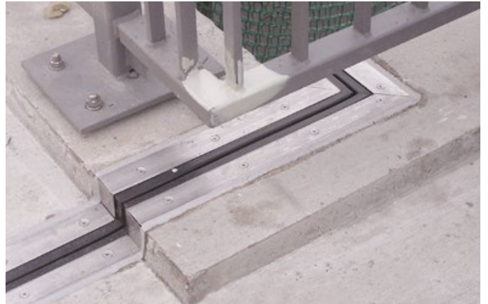
Refurbishment pedestrian bridge, Eilenburg, Germany
